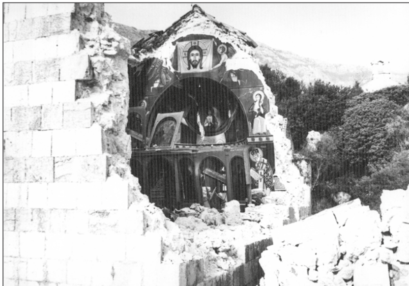
Manastir Gradište / The Gradište Monastery
